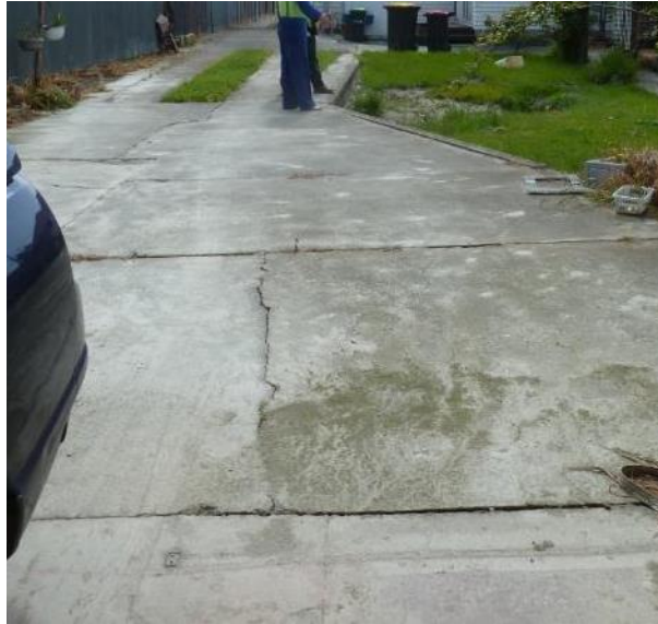
Figure 96: Cracks in the driveway next to Patch C.
