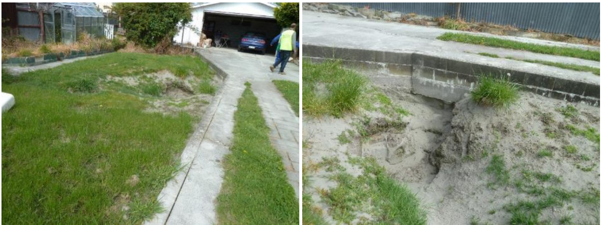
Figure 94: Ground photographs of the sinkhole within Patch C.
